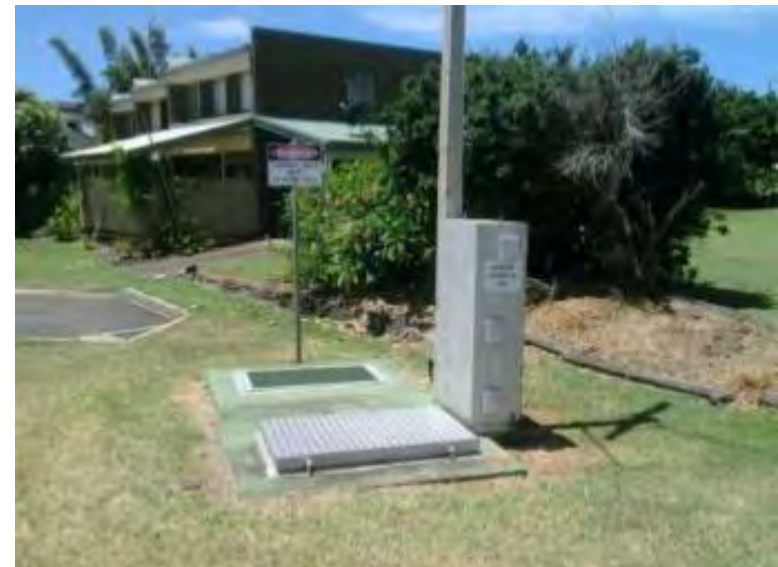
Typical SCADA controlled sewage system
