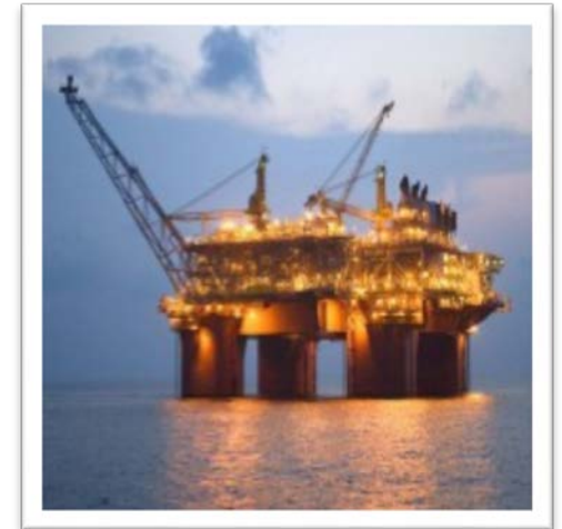
Atlantis Deepwater Oil and Gas Platform; Gulf of Mexico Image Courtesy of Off Shore Technology, http://www.offshore-technology.com
