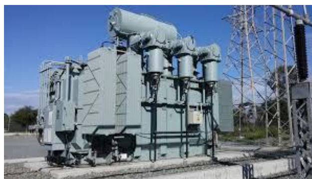
Figure 4 A grid reactor
