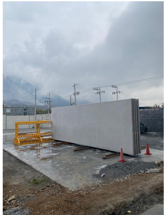
Figure 2: Finished precast concrete wall panels stored at the prefabrication plant prior to transportation and installation.
