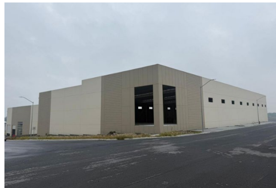
Figure 3: Examples of precast concrete wall panels installed in industrial buildings and perimeter boundary walls.
