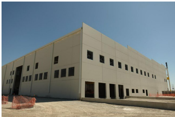
Figure 3: Examples of precast concrete wall panels installed in industrial buildings and perimeter boundary walls.
